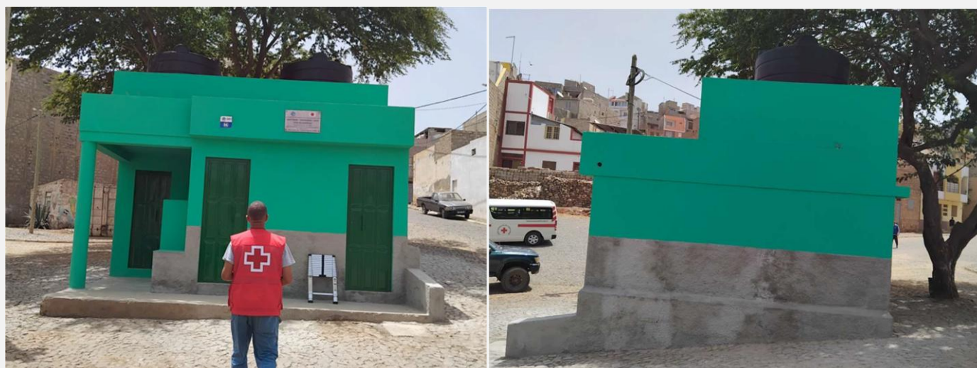
Water sources (sentinas) rehabilitation in progress, in São Vicente, March 2026, Credits: CVCV
